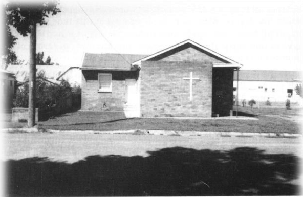
The "new" building after brick veneering.
