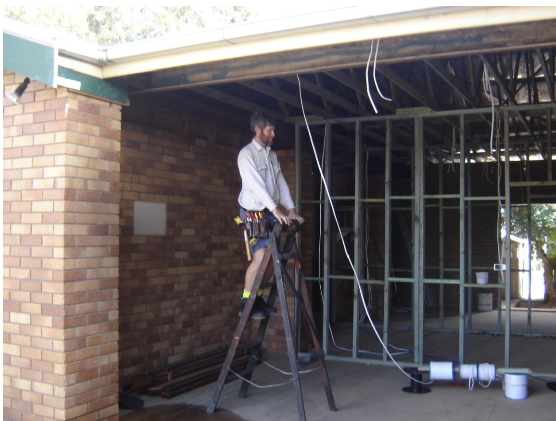
Phil Thring installs electrical cabling in the new foyer.
